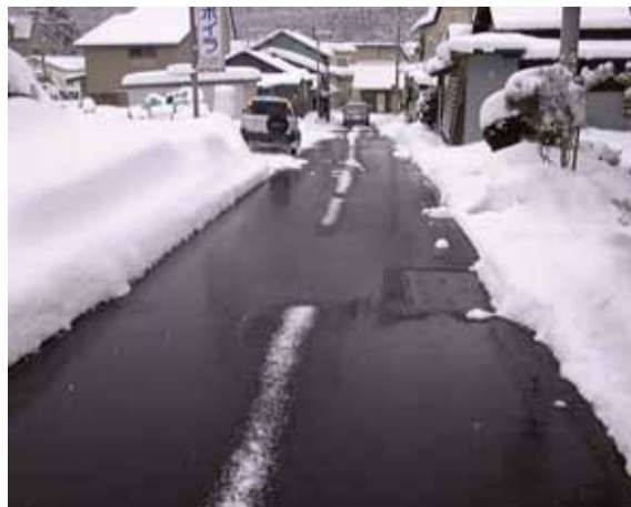
Road snow melting (Kitaakita City, Akita Prefecture)
